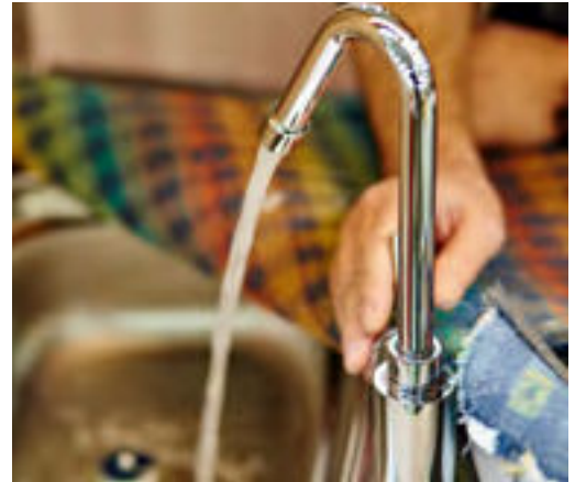
Correct installation of the hydraulic systems.
