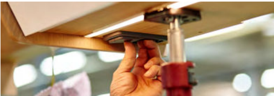
Check on operation and correct installation of the electrical systems.
