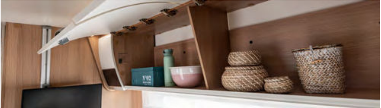
Wall units installed leaving a space from the wall of the motorhome, so that the air is evenly distributed and any condensation or mould is prevented.
